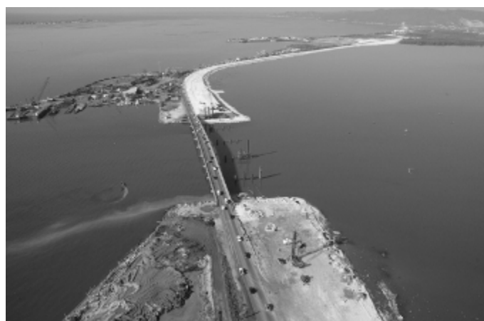
Figure 3. Site works in Jamaica – View of the bridge abutment area
