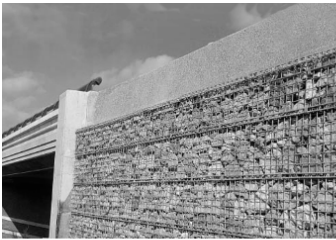
Figure 4. Wire-faced MSE Wall – 1H:4V Wall
