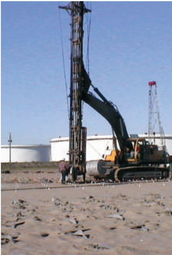
Installing Wick Drains to prepare the ground for the addition of several above ground storage tanks.
