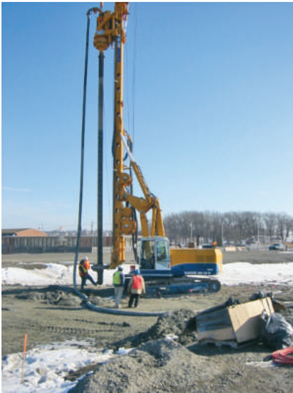
DGI-Menard installed 1,211 Controlled Modulus Columns to depths up to 31 feet deep.
