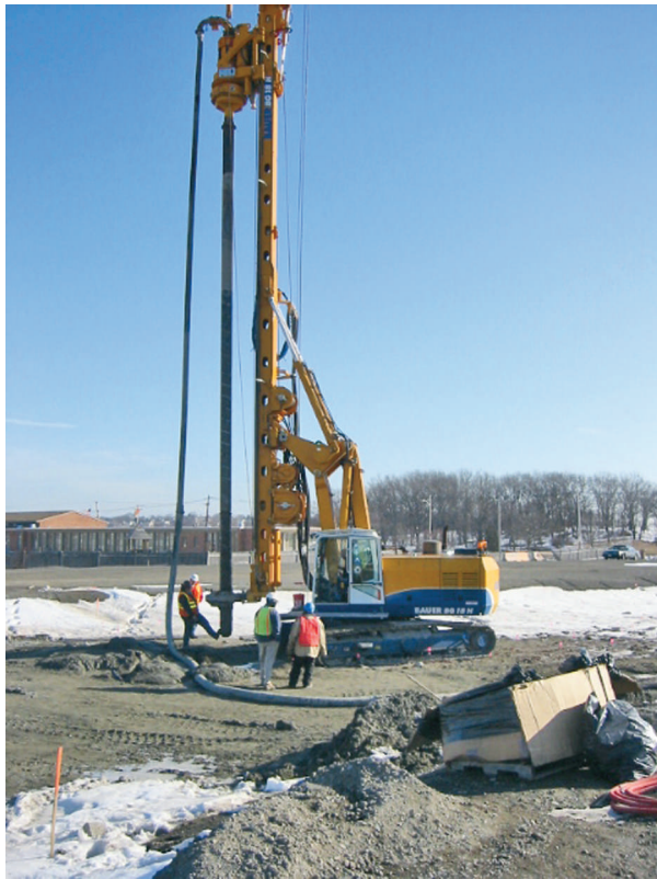
Menard installed 1,211 Controlled Modulus Columns to depths up to 31 feet deep.
