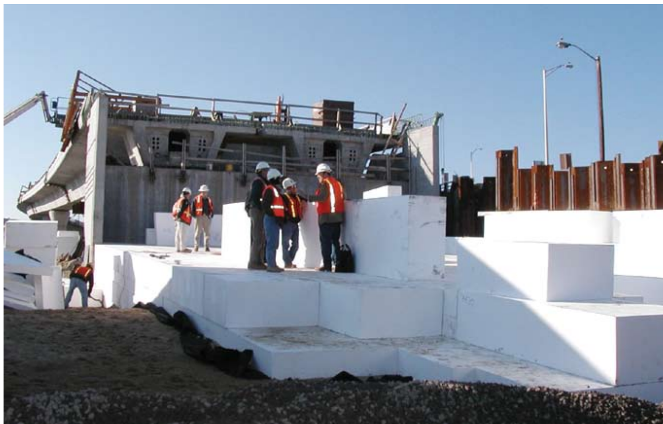
Figure 1. Massachusetts Central Artery/Tunnel embankment fill.
