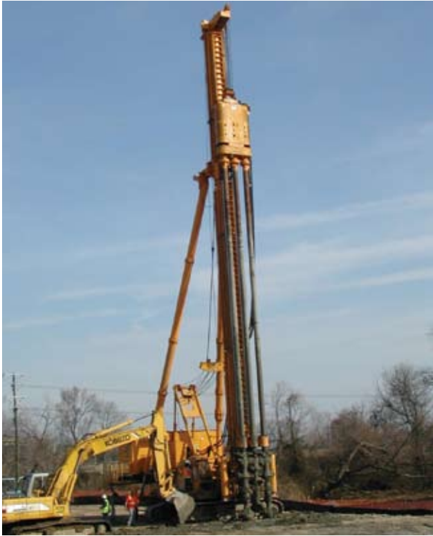
Figure 2. Deep soil mixing rig.
