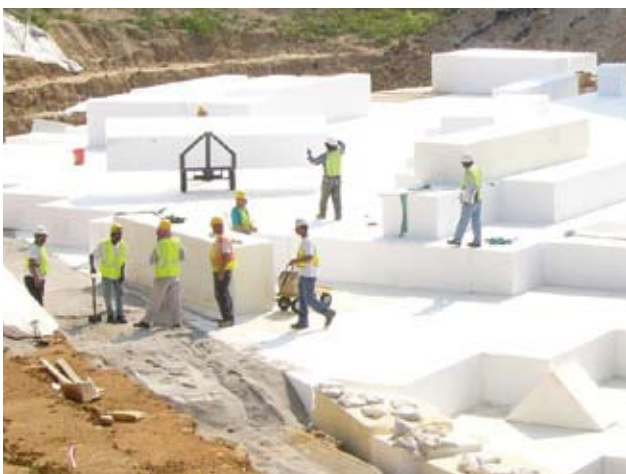
Figure 3. VA Route 1 over I-95 embankment fill.
