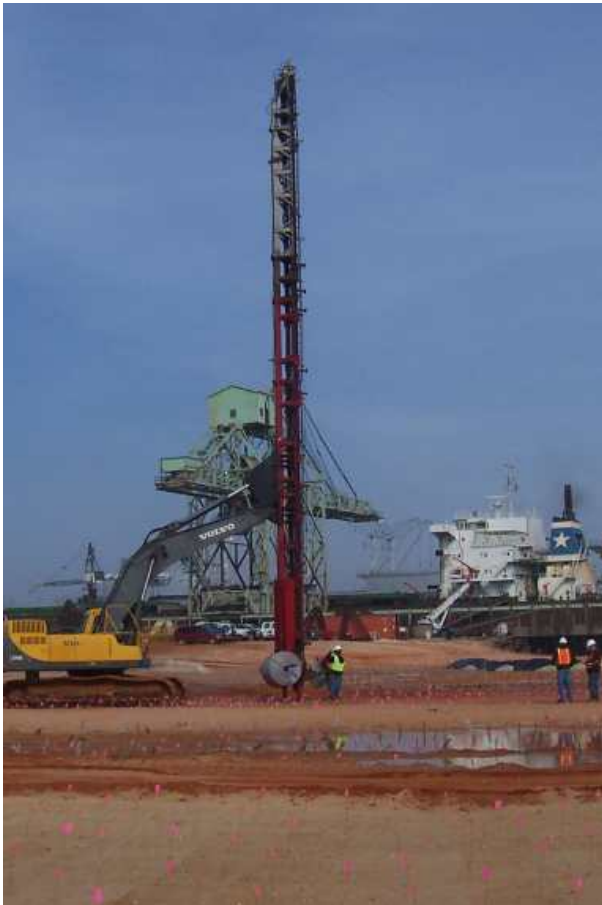
Installing Wick Drains near the port terminal bulkhead
