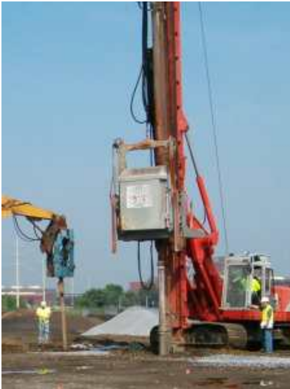
DGI-Menard installed over 1,100 Vibro Stone Columns up to depths of 25 feet.
